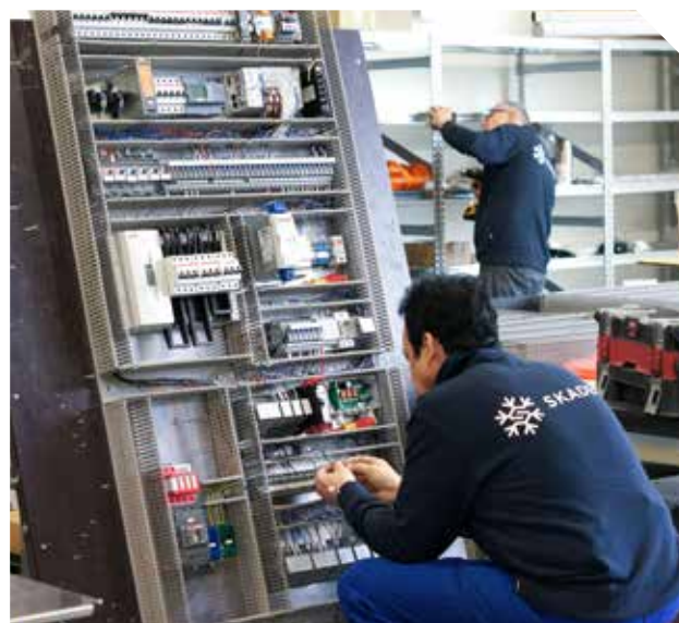
Control cabinet construction
